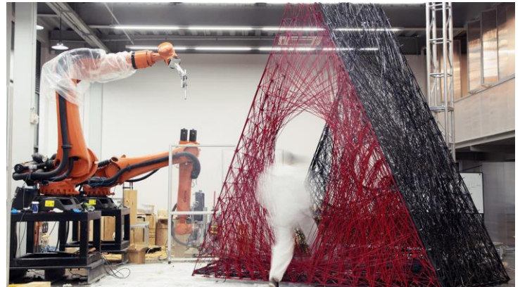
carbon fiber construction process
